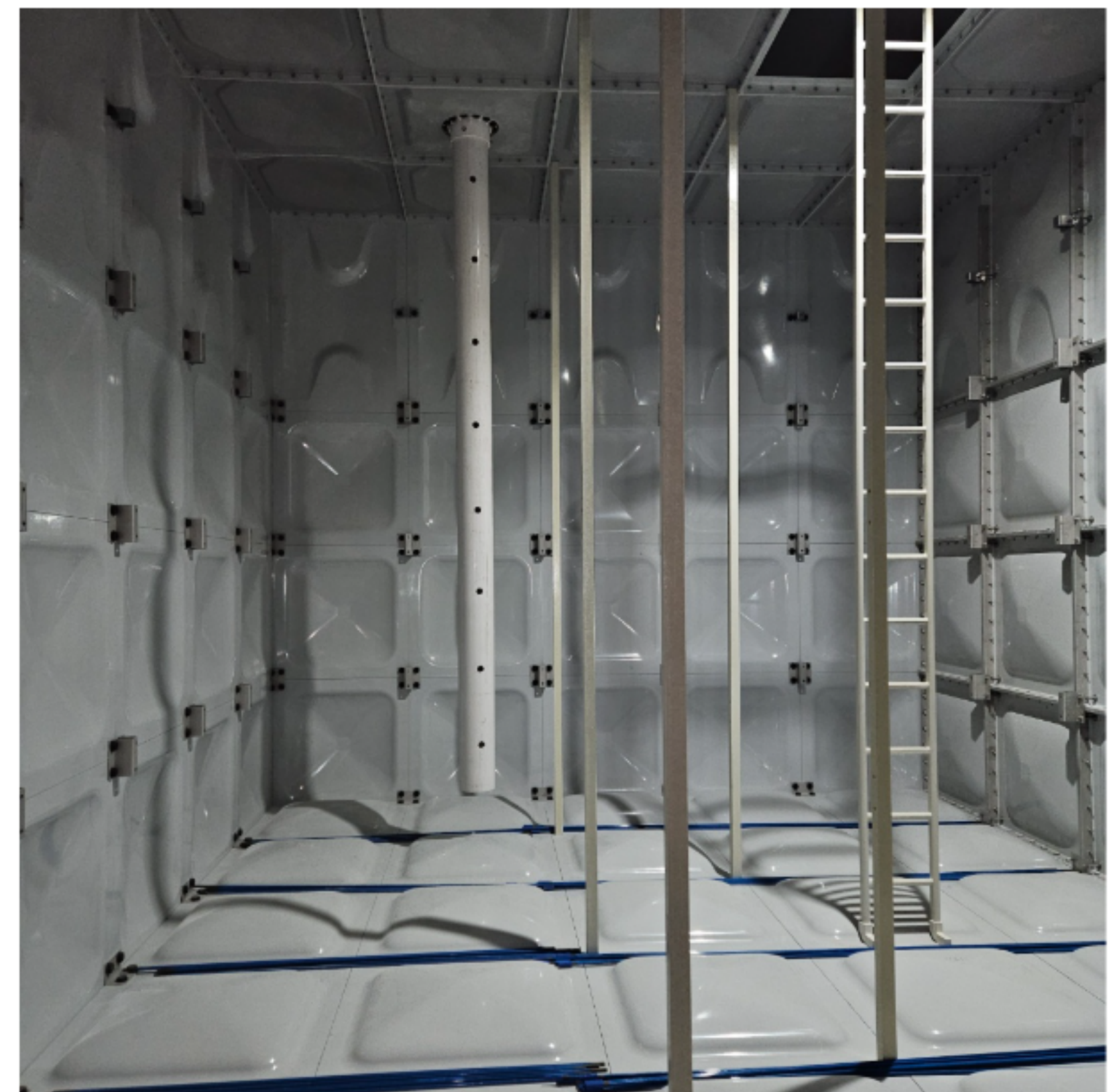
3 Internal Tie-Rod & Roof Support Assembly
