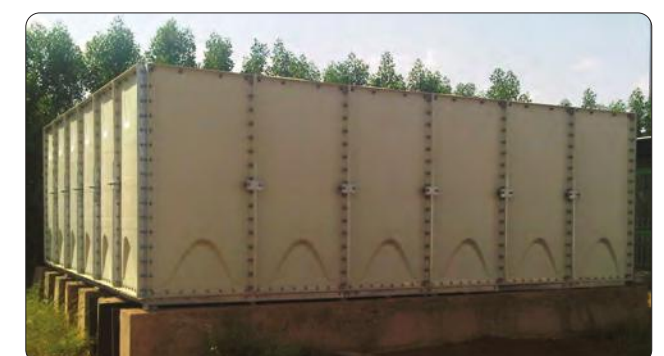
Tank Size 6m x (3+3)m x 2mH : 72 Ton
