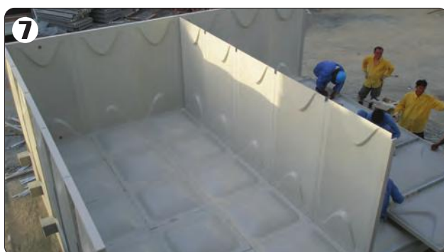
Erect wall and partition panel
