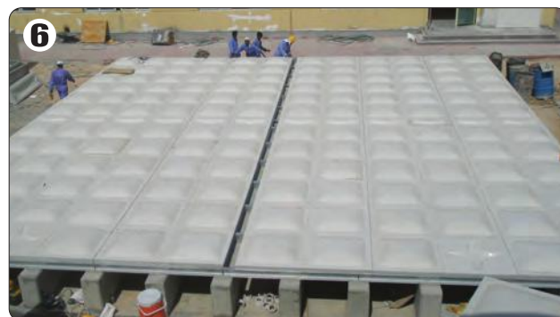
Assemble bottom panel
