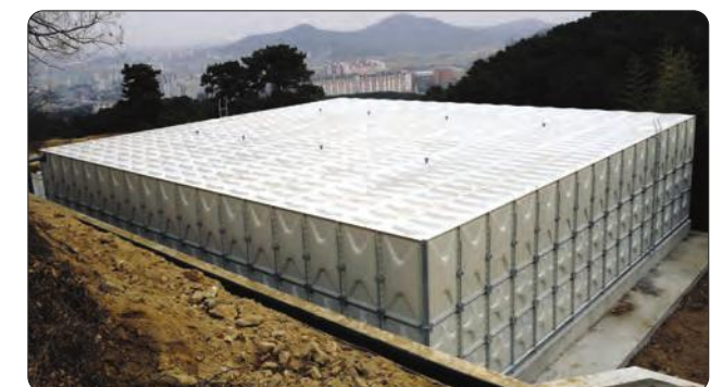
Tank Size 16m x 17m x 4mH : 1088 Ton
