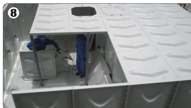
Assemble roof panel and manhole
